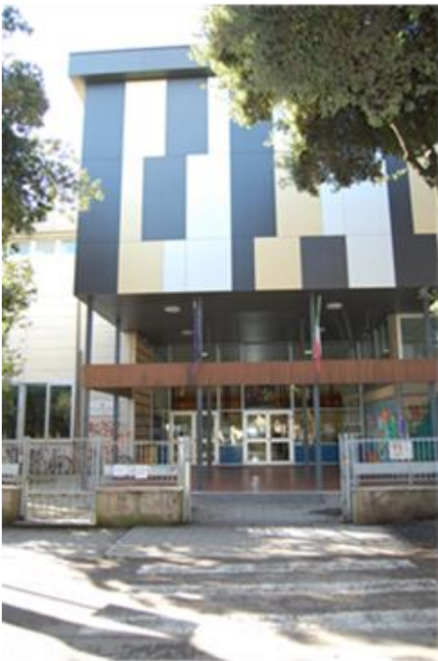
Fig. 12. The main entrance.
