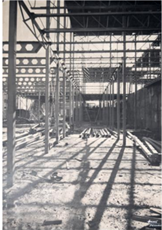
Fig. 3. The original structure in 1964.
