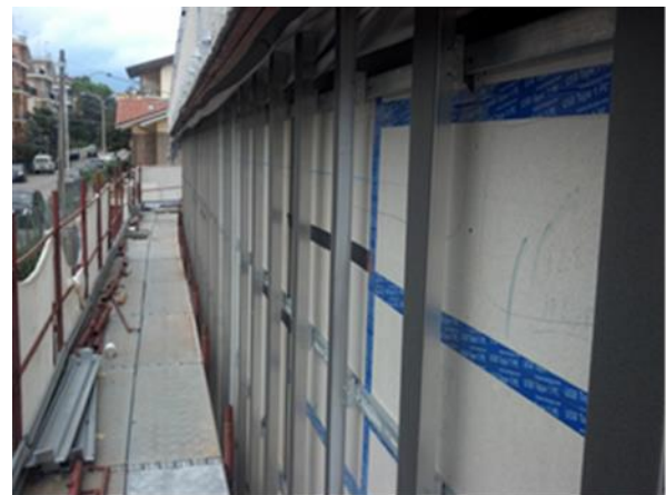
Fig. 8. Ventilated wall structure.
