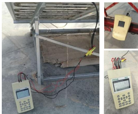
Figure 6: Solar system analyzer and its connection to the PV/T panel
